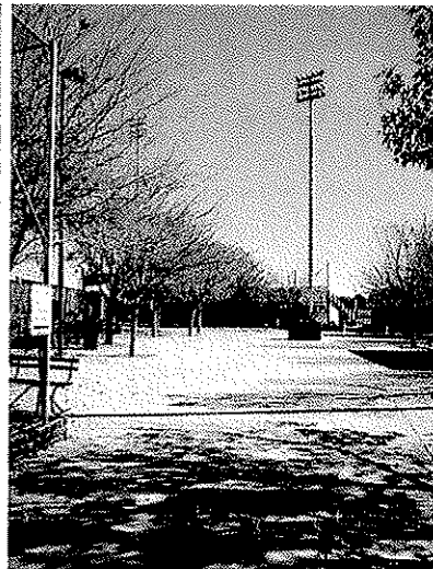
The facility has lighting as well.
