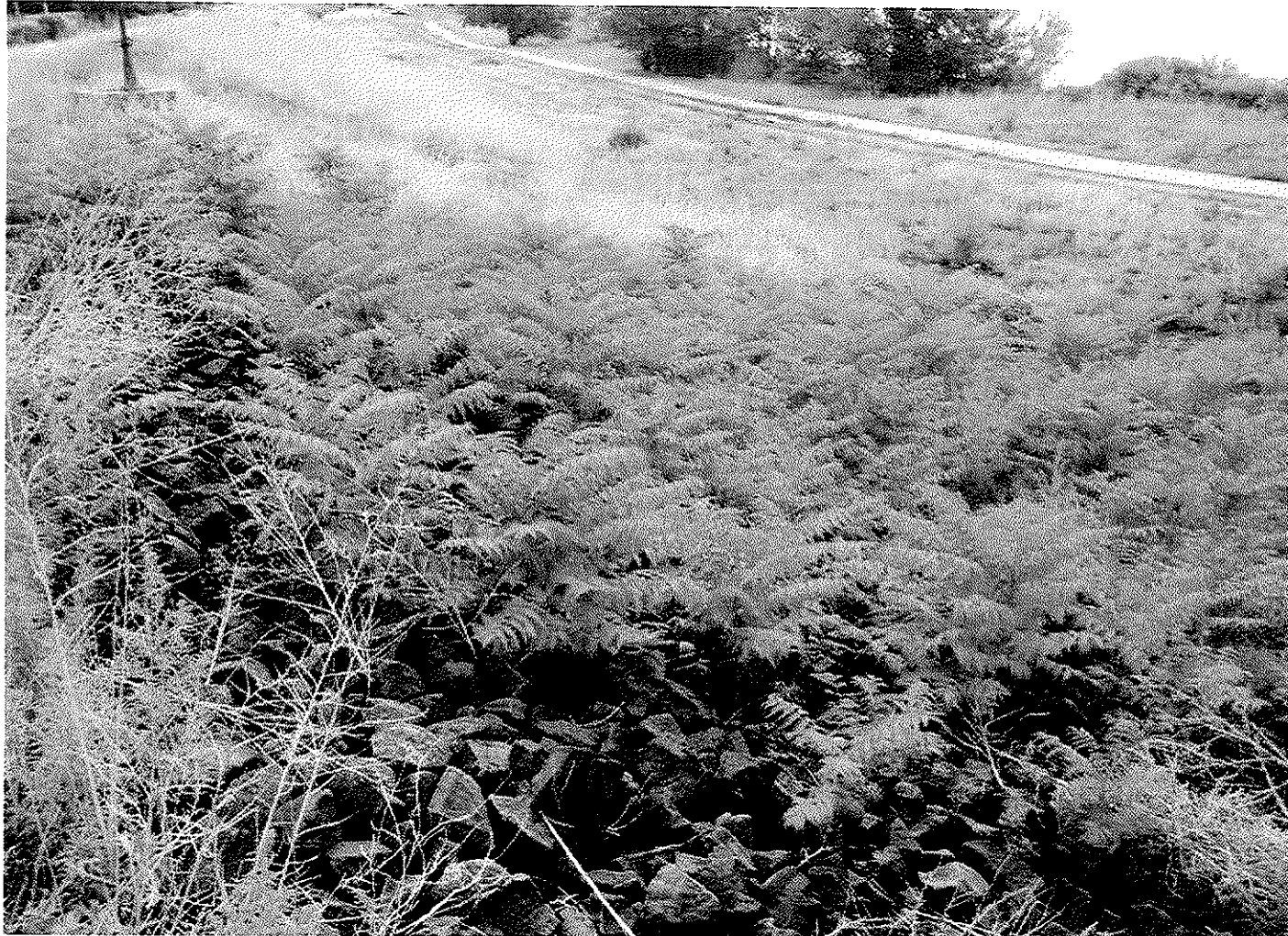
Inspect ID: 0008_2008_a_0005 Name: USACE_CESPA_0008_2008_a_0005_1.jpg Caption: Numerous, small trees growing in rip rap slope protection.
