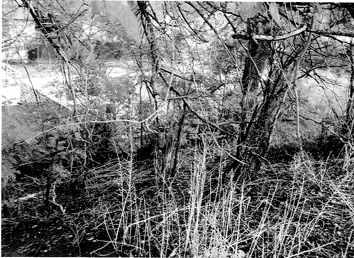
Inspect ID: 0008_2008_a_0006 Name: USACE_CESPA_0008_2008_a_0006_2.jpg Caption: Trees growing at levee.
