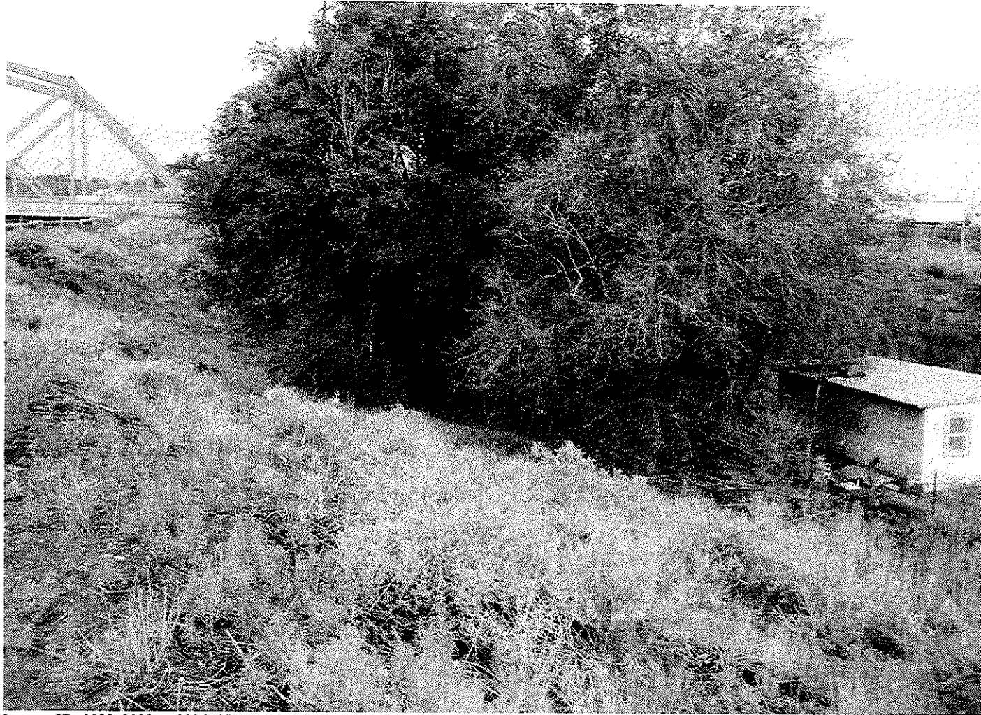
Inspect ID: 0008_2008_a_0006 Name: USACE_CESPA_0008_2008_a_0006_1.jpg Caption: Trees at levee toe.
