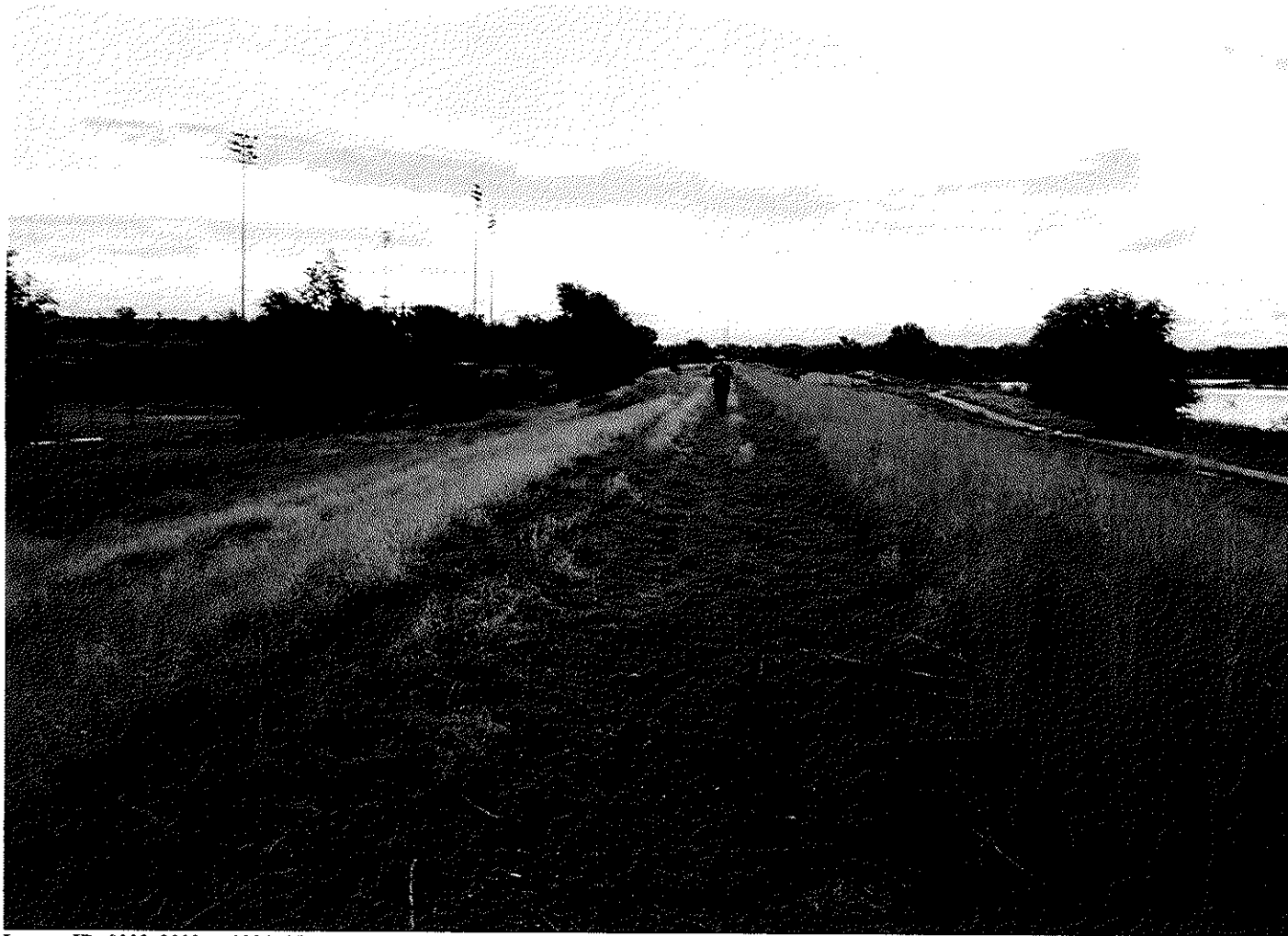
Inspect ID: 0008_2008_a_0004 Name: USACE_CESPA_0008_2008_a_0004_1.jpg Caption: Grass needs to be mowed prior to inspection.
