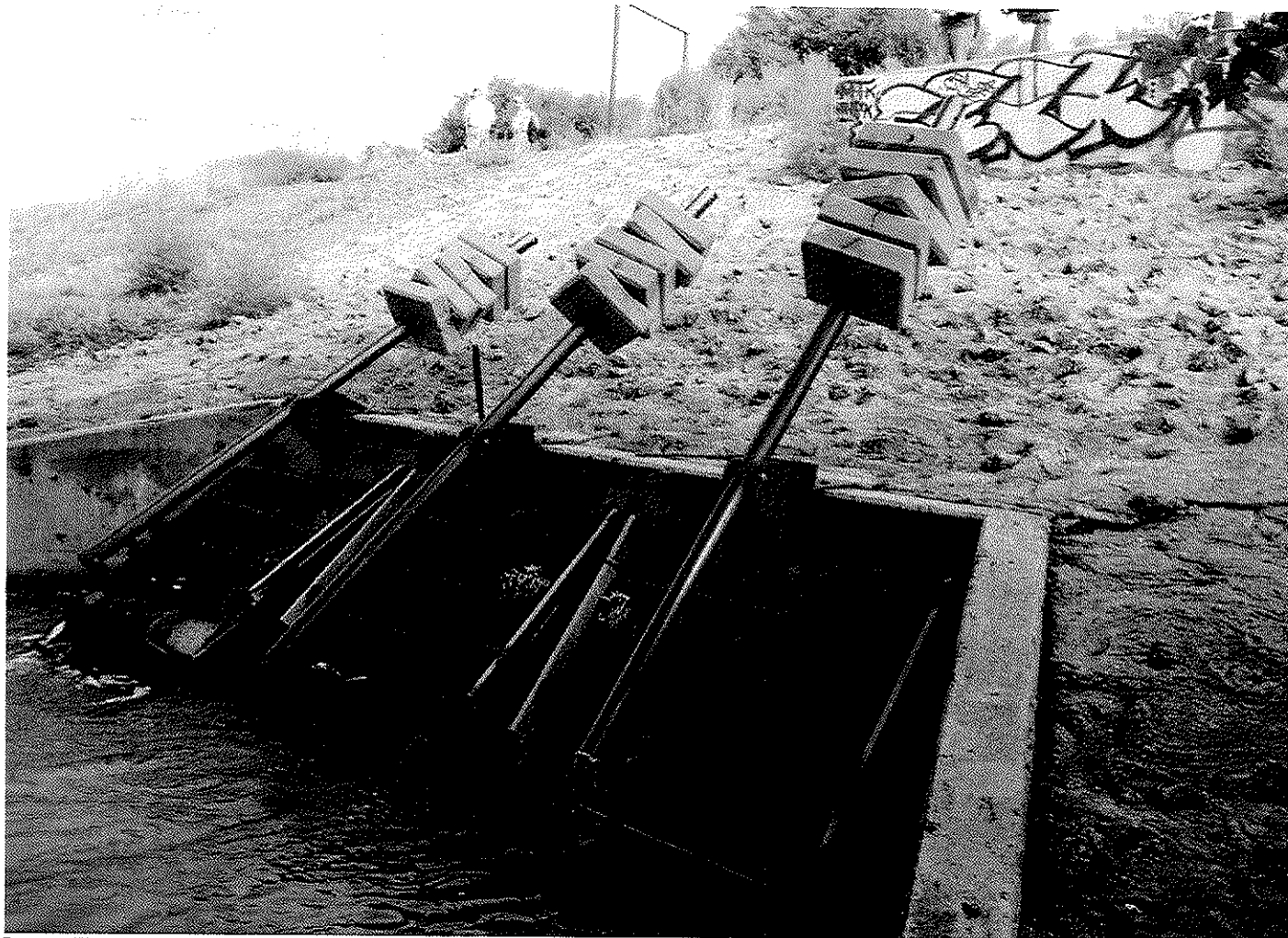
Inspect ID: 0008_2008_a_0002 Name: USACE_CESPA_0008_2008_a_0002_1.jpg Caption: Flap gates at drainage structure.
