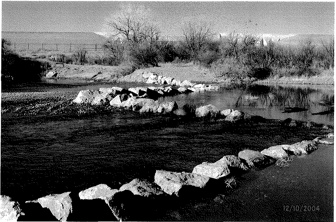
W-Weir Constructed in River Adjacent to Fish Hatchery Ponds
