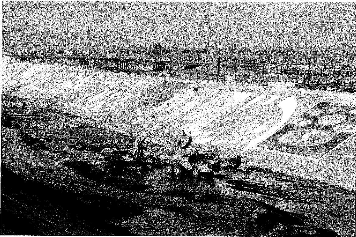
Constructing Drop Structure No. 6 Along Levee
