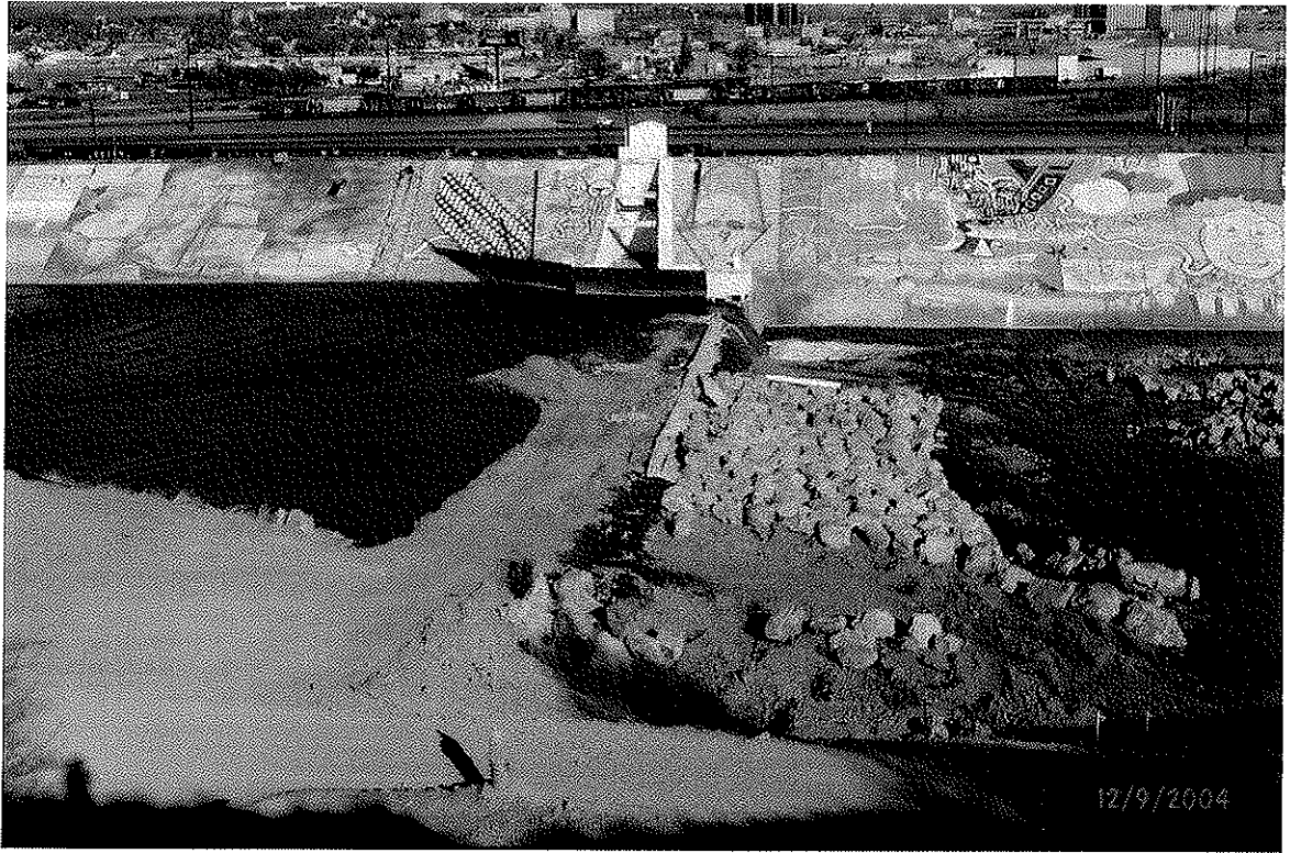
View of Aquila Dam and Drop Structure No. 1 Under Construction
