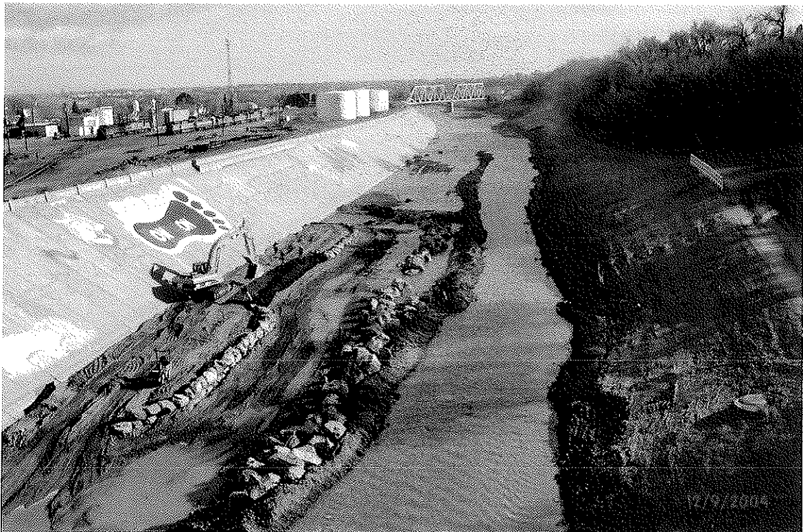
Looking Southeast from Main Street to Santa Fa Avenue
