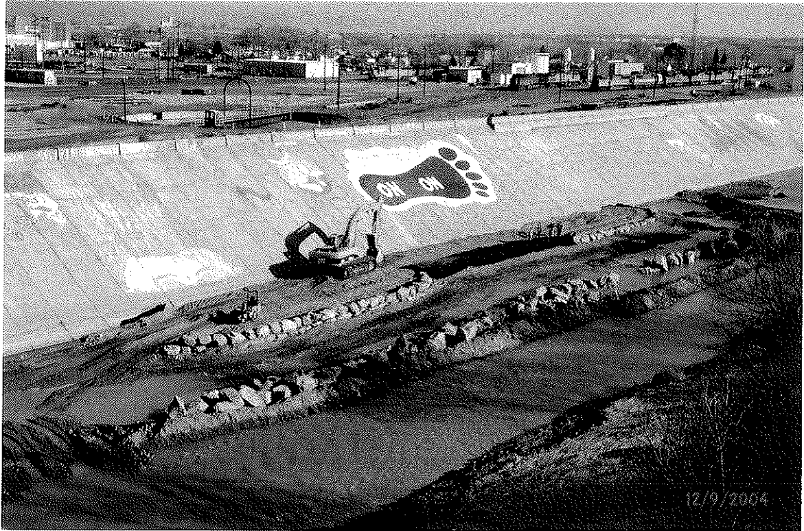
Vegetated Bar Construction Southeast of Main Street
